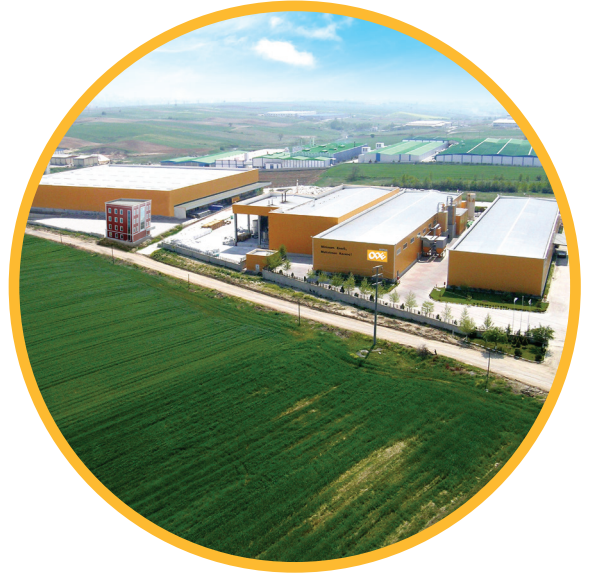
ODE Çorlu/Tekirdağ, Turkey Production Facilities
